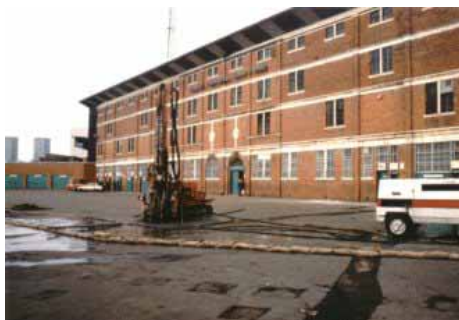
Drilling and grouting at the Celtic Football Ground, Glasgow
