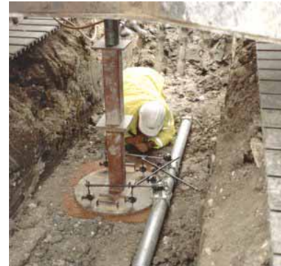
A plate loading test.
