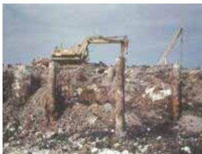
Reclaiming the site of the former chemical works, Ilford, east London
